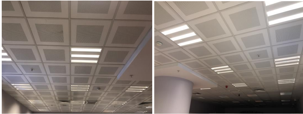
Figure 22: The ceiling images Office A (Author Archive)
