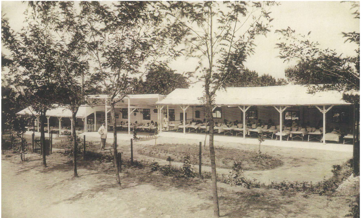
Figure 3.1.2.7. Conversion of the ateliers to the preventorium's outdoor cure areas. (Source: Kolay & Memiş, Talebe Tedavi Yurdu'ndan Öğretmenler Hastanesi'ne, 2017d)
