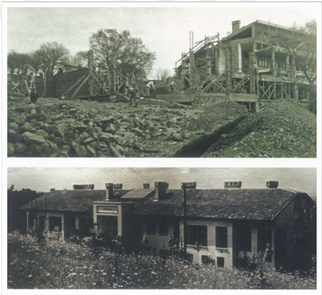
Figure3.1.2.8. During the construction of additional sanatorium buildings. (Source: Kolay & Memiř, Talebe Tedavi Yurdu'ndan Öğretmenler Hastanesi'ne, 2017d)
