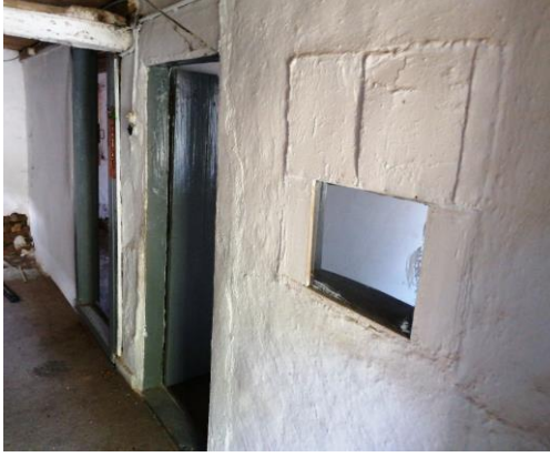
ġekil 3. 69 Ortak aydınlatma niğ ıġıklık, E134, (Doġan Talyak, 2021)
