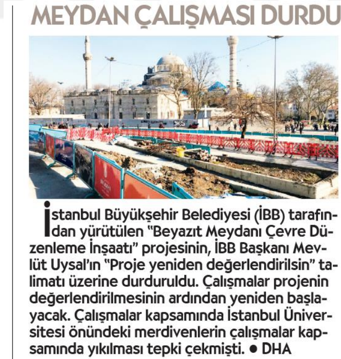
Figure 3.36.: Work for square has stopped 47 (Cumhuriyet, 02.03.2018)
