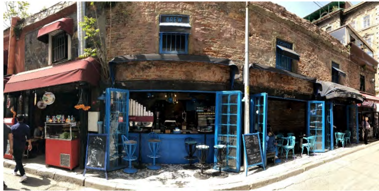
A new generation café named Brew Café in the historical structure (Letter F on Key Map) (Akbaş,2019)
