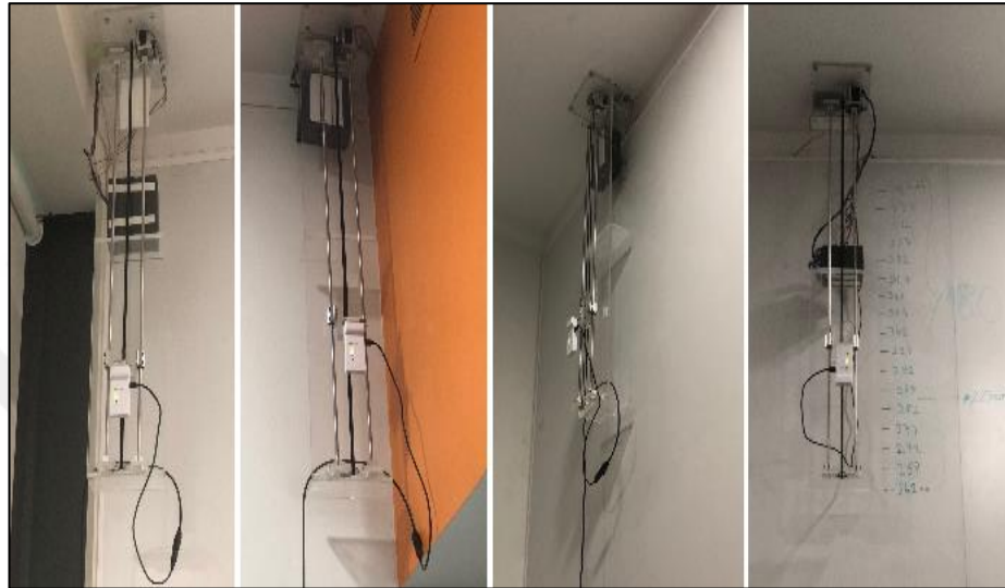
Figure 3.2 Ceiling installation of the anchors.
