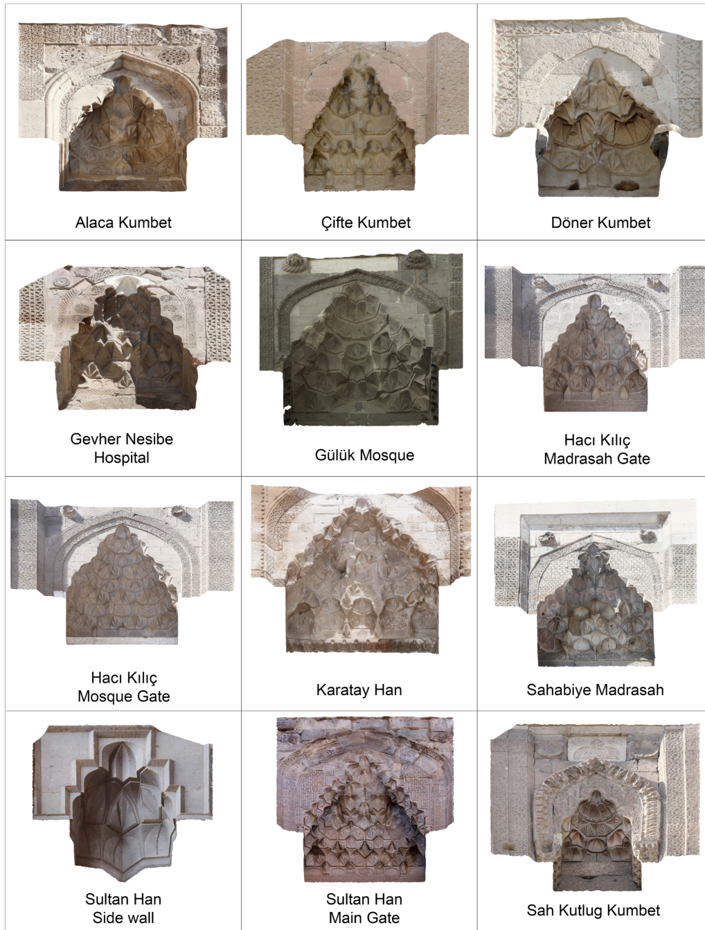
Fig. 4. The photogrammetric models of 12 muqarnas structures produced in Agisoft.
