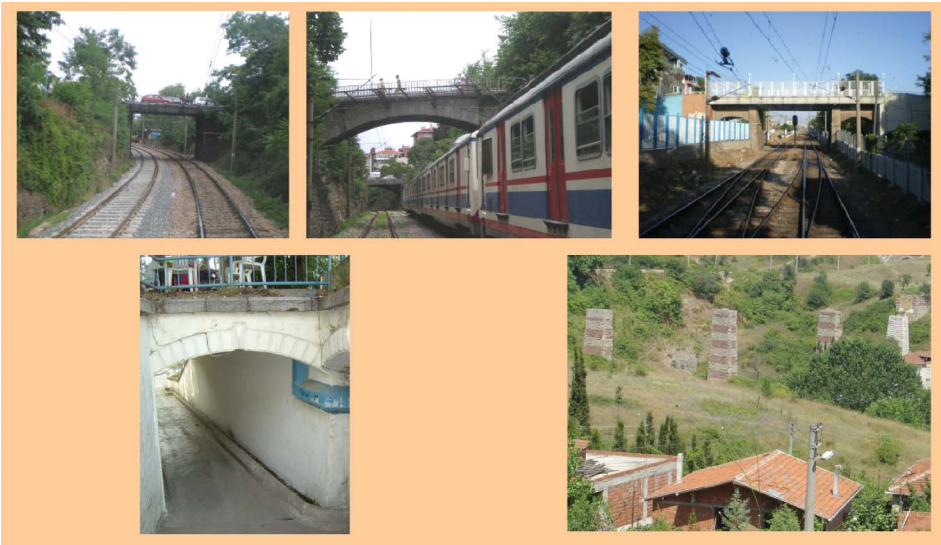
Figure 5. Photographs of some of the historic bridges (color figure available online).
